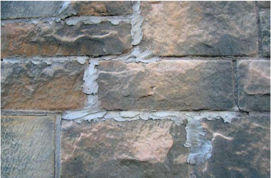
*Poorly executed repairs in portland cement*
