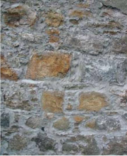
*Poor quality cement pointing can have a poor visual impact*
