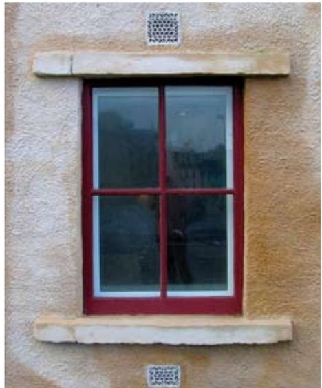
*Lime drying out quickly after heavy rain*
